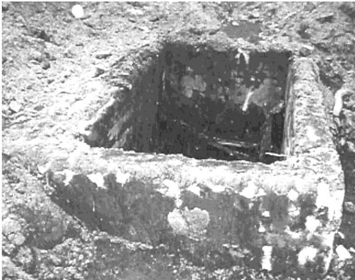
Fig. 3: Concrete tar separator box discovered during site remediation at Dover, New Hampshire. The box measures about 2 x 3 m in plan (Courtesy of New Hampshire Department of Health Services, Concord, N.H., 2002)
